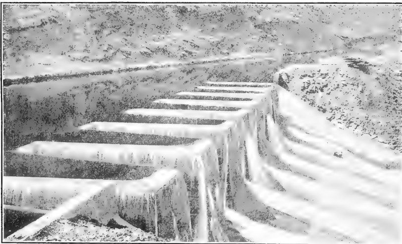
FIG. 2.—SPILLWAY WITH CONCENTRATED CREST LENGTH, KLAMATH PROJECT, OREGON.
